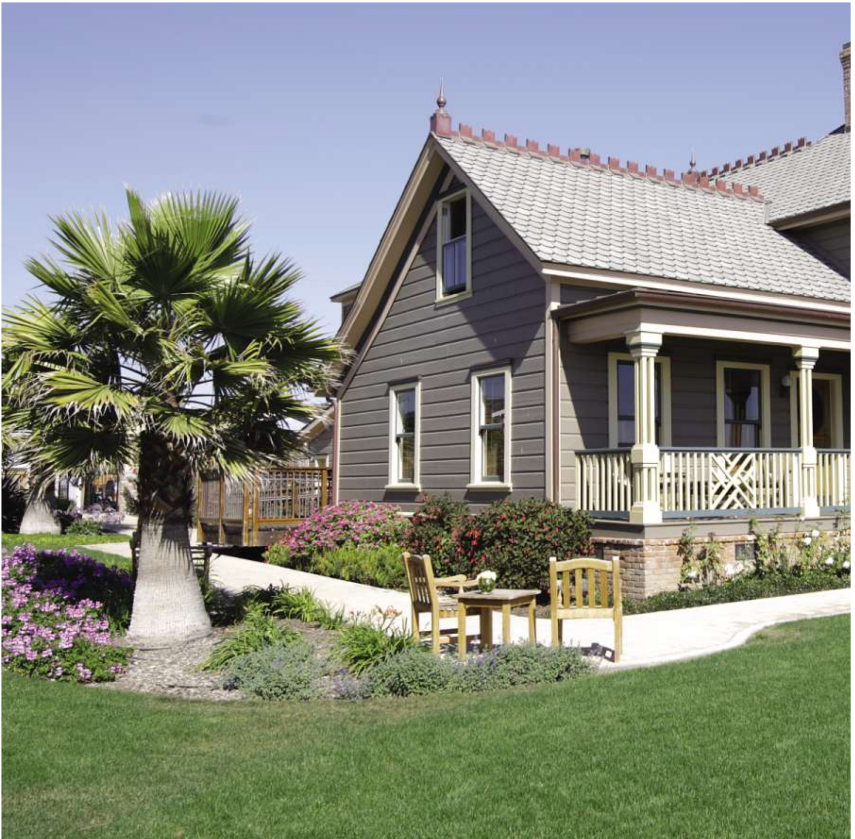
THE STATELY VICTORIAN CASS HOUSE , built in 1875 by Cayucos founder Capt. James Cass, has been sensitively renovated and turned into an English-style inn by Gary and Nancy Bagnall. Landscape design was by Firma of San Luis Obispo.
